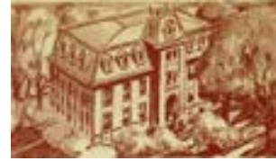
MORRILL HALL, OLDEST ACADEMIC BUILDING STILL IN USE, CONSTRUCTED
