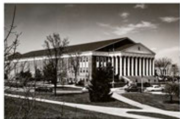
RECKORD ARMORY OPENS
